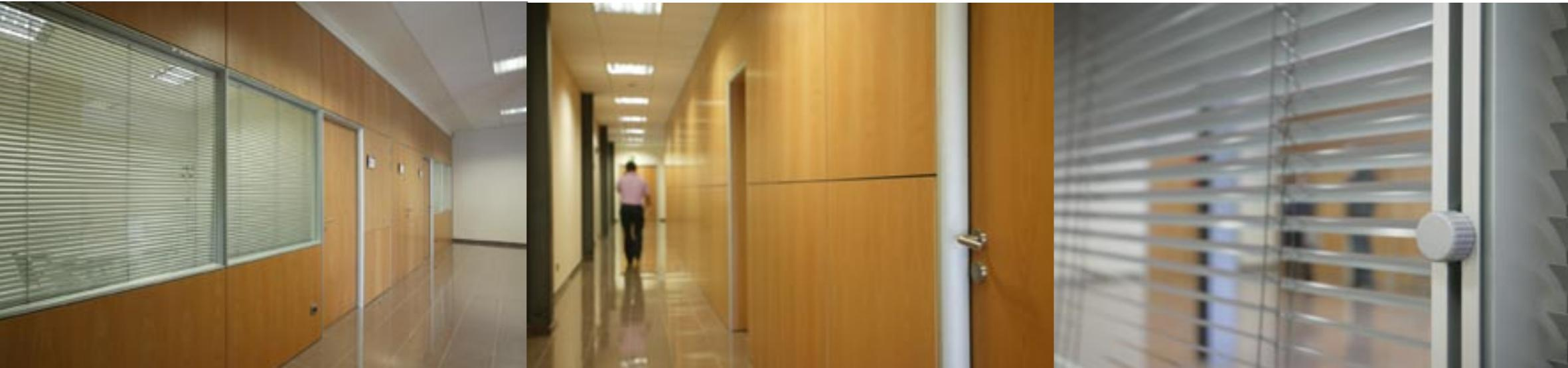
The spaces separated with glass-fitted modules can ensure privacy by installing adjustable-opening Venetian blinds between the panes.
